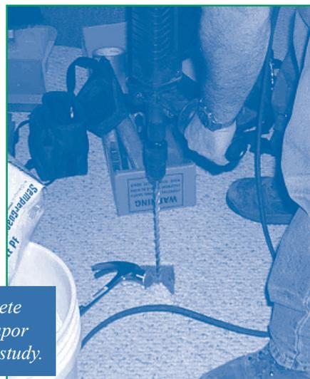
**Figure 2.** Only a small hole in the concrete slab was needed to install a multi-use vapor probe in each basement of the Raymark study.
