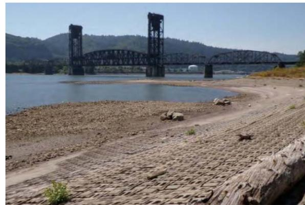
Figure 2. Exposed ACB and sand cap armoring at the McCormick & Baxter site.
