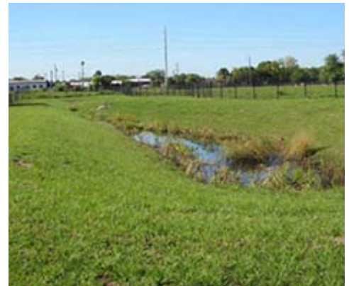
Figure 1. A stormwater retention pond at the Sanford site for mitigating soil erosion.
