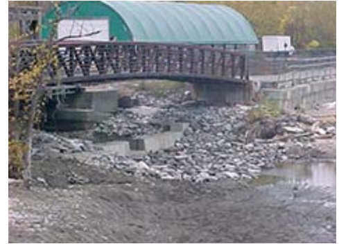
Figure 2. 50-foot weir at the Pine Street Canal outlet.
