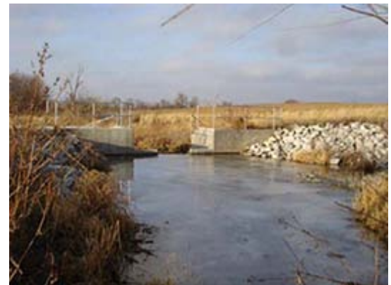
Figure 3. 12-foot-wide drop structure controlled by a 5-foot-wide stop-log system at the Murdock Groundwater Plume site.
