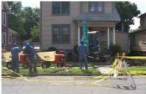
Residential cleanup of hazardous waste
