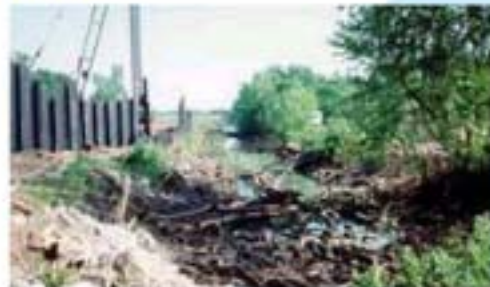
The East Ditch, located at the south end of Bowers Landfill in Ohio, contained discarded tires and debris
