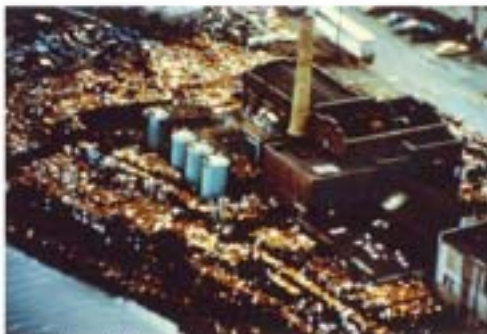
Abandoned chemical warehouse in Elizabeth, New Jersey
