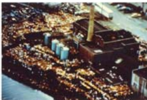
Abandoned chemical warehouse in Elizabeth, New Jersey
