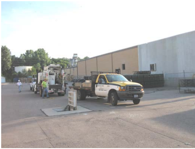
1 HCS Well Recovery Well Vault Exterior.
