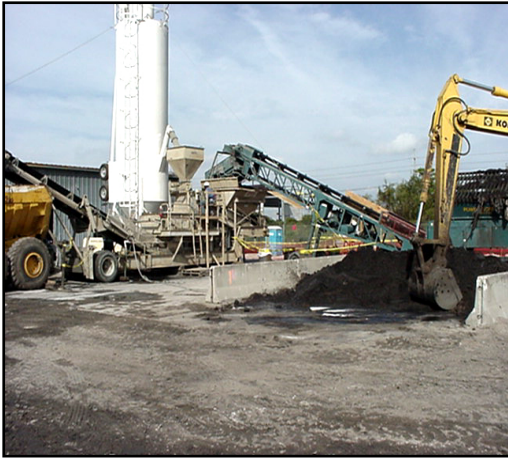
Figure 3-2. Ex-Situ Soil Mixing at the Peak Oil Site
