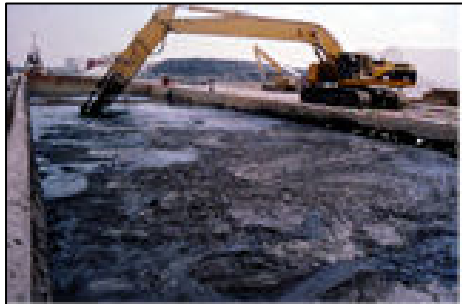
Figure 7-5. Dredged Sediment Undergoing Treatment in Barge
