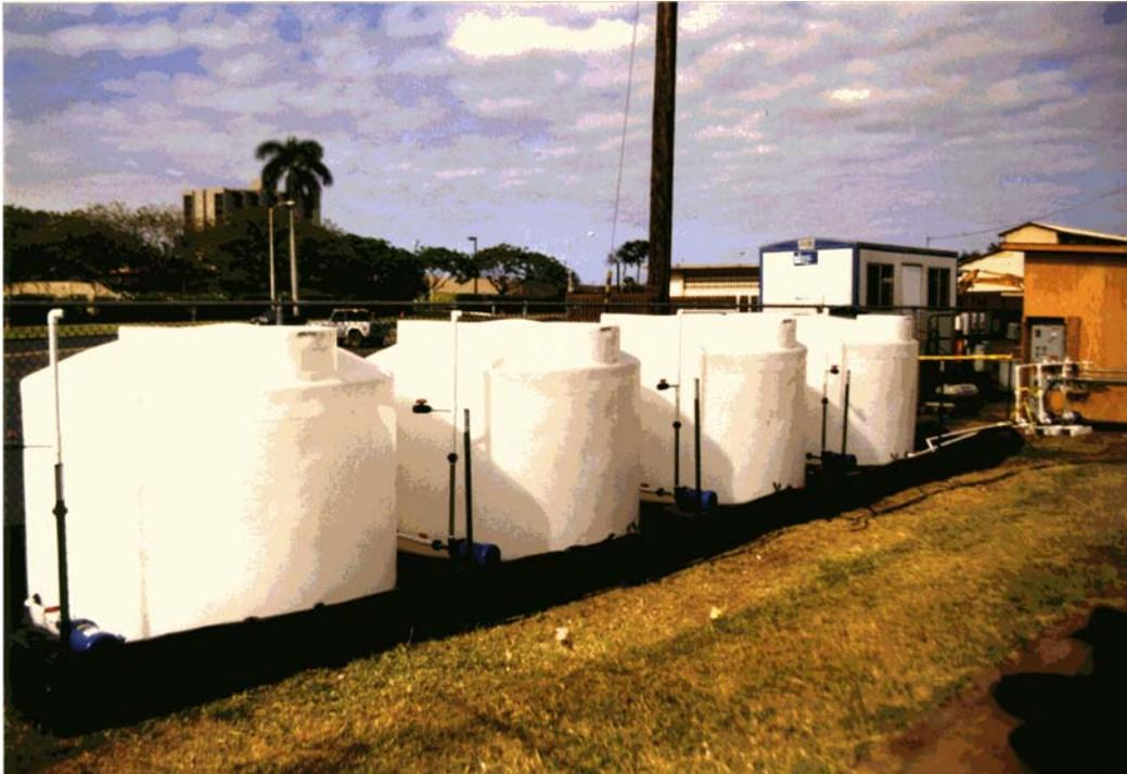
**Figure 3-1. HDPE Storage Tanks Used for Blending Electrolyte Solutions**
