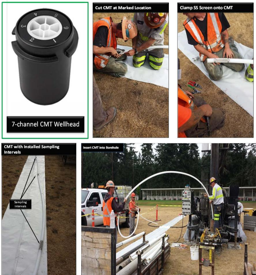
**Figure 10. CMT well installation during field demonstration.**
