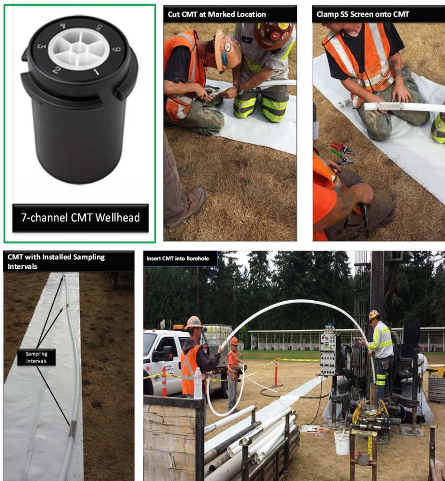
**Figure 10. CMT well installation during field demonstration.**
