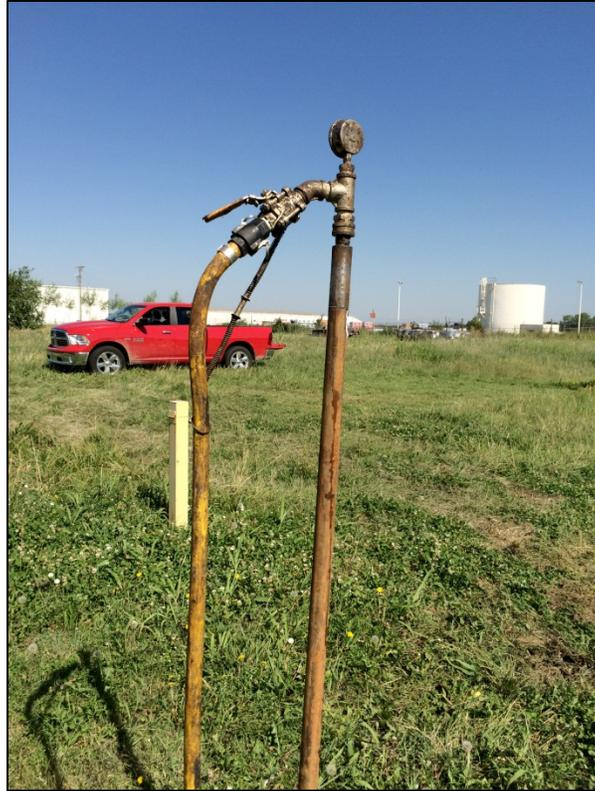
Photo 11: EHC injection rod with hose connected to injection manifold.
