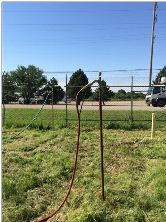
Photo 12: EHC injection rod with hose connected to injection manifold.
