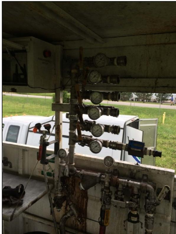
Photo 8: Injection manifold.
