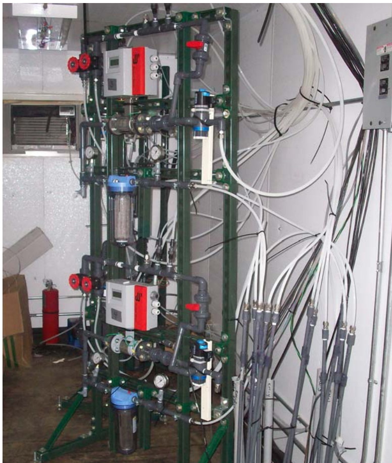
Figure 5-19. Photograph of Amendment Injection Rack
