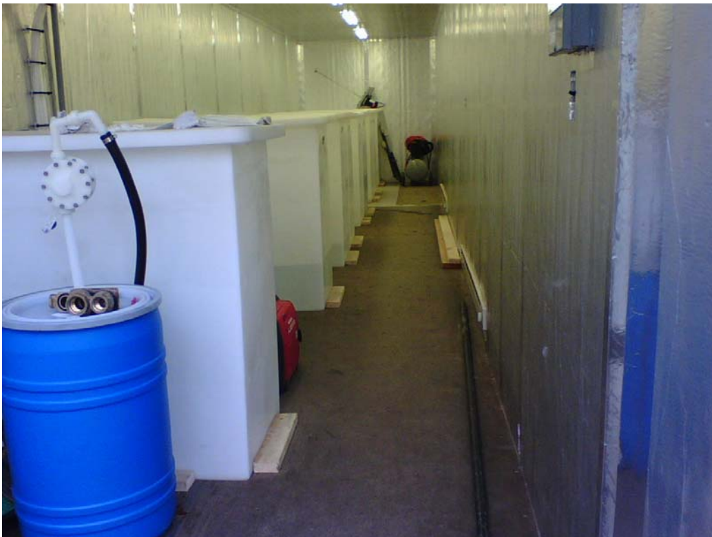
Figure 5-18. Photograph of Buffer Tanks in 40-foot Conex Box
