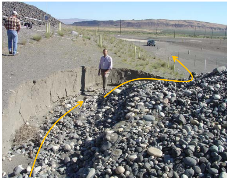
Figure 3.22. North-facing photograph taken on June 16, 2004. The orange lines indicate the path and direction of the runoff water in May 2004 after severe thunderstorms.
