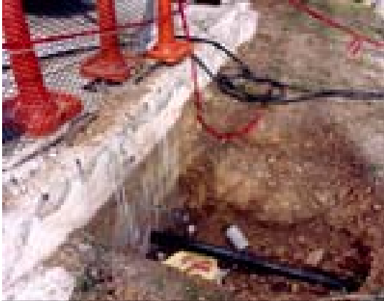
Entry area for the horizontal drill under a slab
