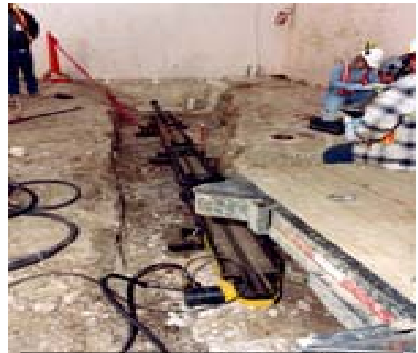
Environmental sampling at the drill site
