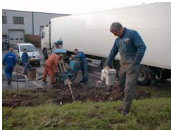
Exhibit A-21. Walkover Locator Receiver In Use
