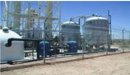
Figure 1.-Typical Above Ground Treatment Technology
