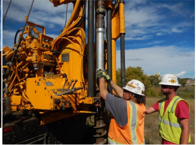
m. Attach the auger string to the drill rig and advance the drill string 2 to 5 feet, depending on the length of core desired.
