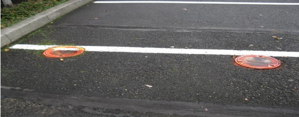
**Photo 11:** Groundwater Monitoring Wells W85-5A and W85-5B identified for decommissioning
