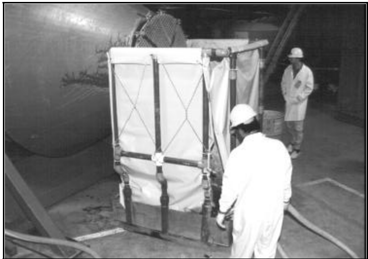
Figure 4. Removing treated soil from the RBR.
