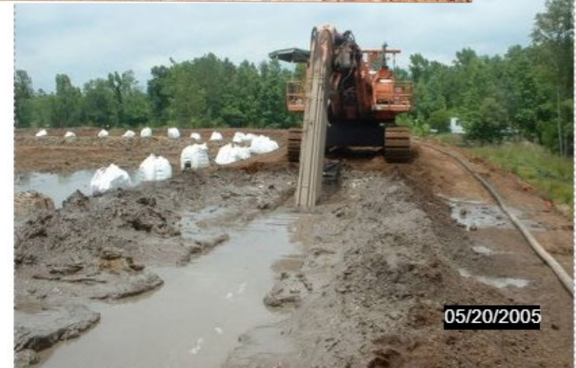
Trenching Near Station 19+00 Heading North of Site
