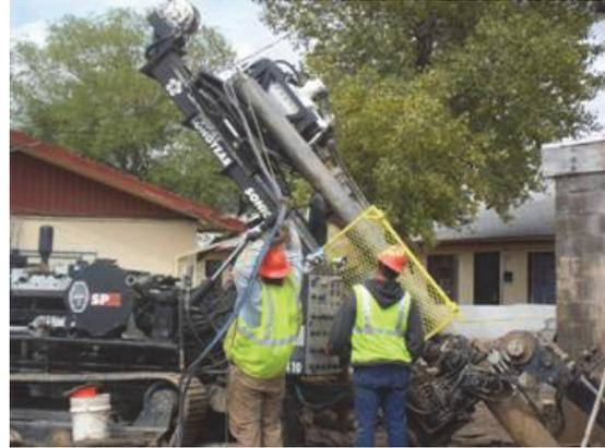
**Figure 6. Sheet pile Electrode Installation**
