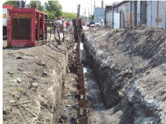
**Figure 7. Horizontal Electrode Installation**
