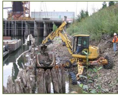
All heavy machinery deployed for removal of petroleum HC-contaminated soil at the Terminal 4 portion of the Portland Harbor Superfund Site in Oregon has used ULSD in advance of federal requirements.
