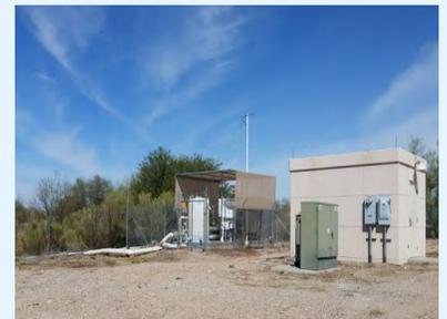
An SVE system with four extraction wells began operating at the Airport Property portion of the Tucson International Airport Area Superfund Site in 2008. The system operates in conjunction with long-term extraction and treatment of groundwater. Vapor-phase GAC adsorption is used to treat the extracted vapors. Since SVE startup, optimization has included:
