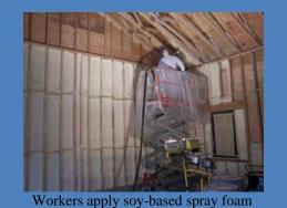
Workers apply soy-based spray foam insulation that acts as a climate barrier and noise reducer.
