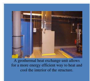
established for the extraction and treatment of groundwater. Prior to going through the treatment process to remove VOC contamination and following sediment filtration, water is carried to a geothermal heat exchange. This unit utilizes the constant temperature to provide a more efficient way of heating and cooling the support areas of the facility (i.e. offices, restrooms, meeting room, etc.).
