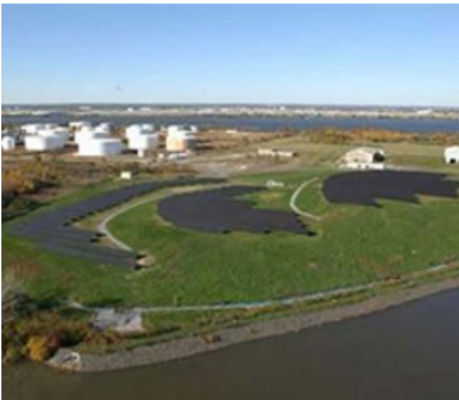
Solar Field in Former Infrastructure: Integrated cleanup and reuse planning allowed installation of the solar field without disruption to tank and building demolition or to operation of large-scale groundwater P&T and SVE systems.
