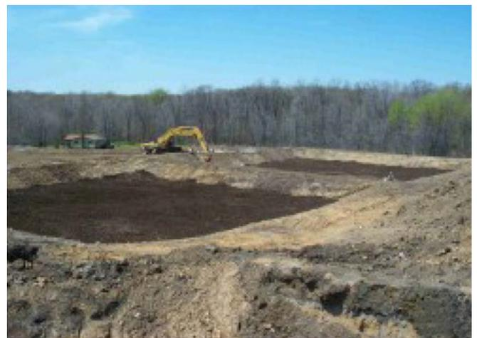
**Compost in Vertical-Flow Pond:** About 6 inches of spent mushroom compost is placed atop limestone in vertical-flow ponds.
