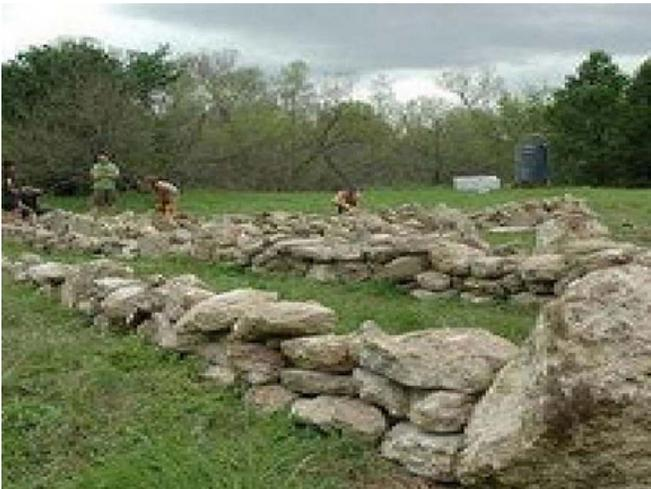
**Concrete Reuse:** Onsite garden beds are constructed of scrap concrete that was salvaged during cleanup.
