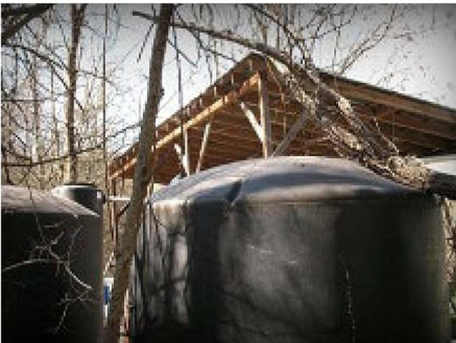
**Rainwater Harvesting:** Rainwater captured from an elevated platform is stored in four tanks, each holding 2,500 to 3,000 gallons, to meet non-potable water needs.
