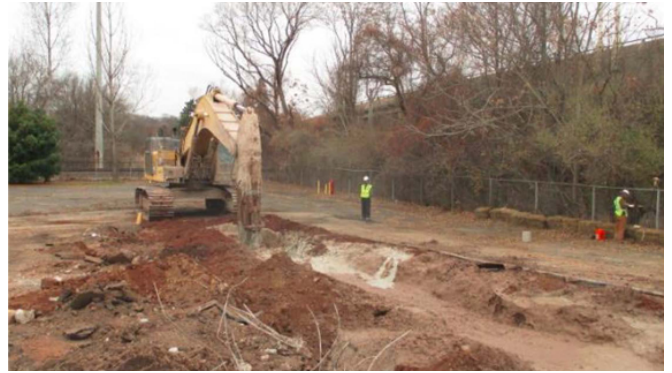
Hydraulic Barrier Installation: The slurry used to construct the hydraulic barrier wall consisted of a 3:1 mix of blast furnace slag and Portland cement. The wall extends to an average depth of 17 feet and is keyed into underlying clay.
