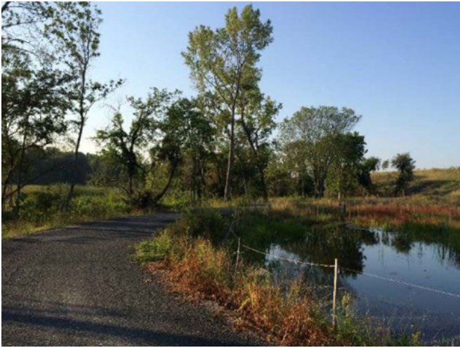
Perimeter Trails: Trails along the ecological preserve's perimeter were constructed above the path of the subsurface hydraulic barrier wall, which is anticipated to remain in place indefinitely.
