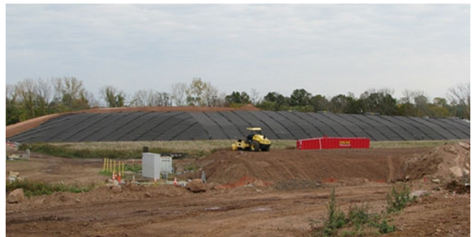
Cover Construction: The reuse of excavated soil to grade the surface beneath constructed covers significantly reduced the need to import clean fill from offsite sources.
