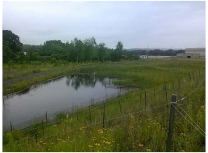
Stormwater Management: Stormwater shed from the cover systems flows to tiered wetlands that were constructed above the water table. A geosynthetic liner at the bottom of each constructed wetland additionally prevents contact between stormwater and contaminated groundwater.
