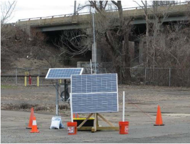
Solar-Powered Monitoring: Portable photovoltaic panels directly powered the air monitoring equipment deployed during corrective measures implementation.
