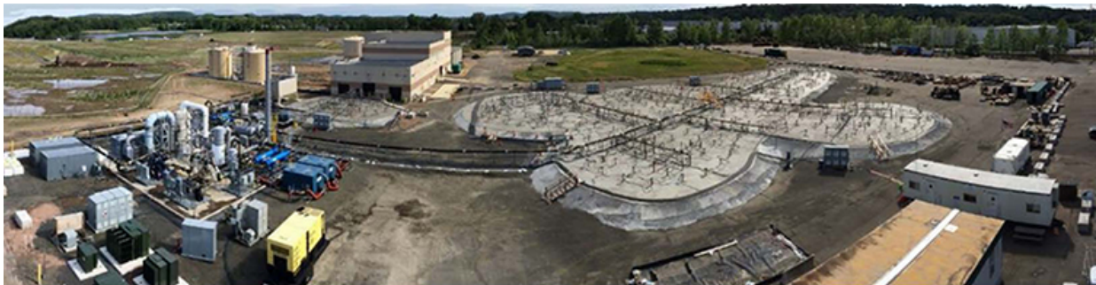
Full-Scale ISTR: The full-scale ISTR system covered two areas occupying approximately one acre.
