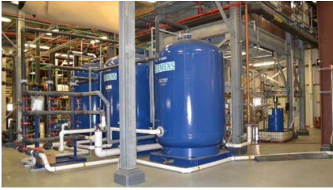
Groundwater Treatment Plant: The extracted groundwater is conveyed to the onsite groundwater treatment plant where it is treated via a biological process to remove volatile and semi-volatile organic compounds, a solids removal system, and UV light and peroxide to remove recalcitrant compounds such as 1,4-dioxane.
