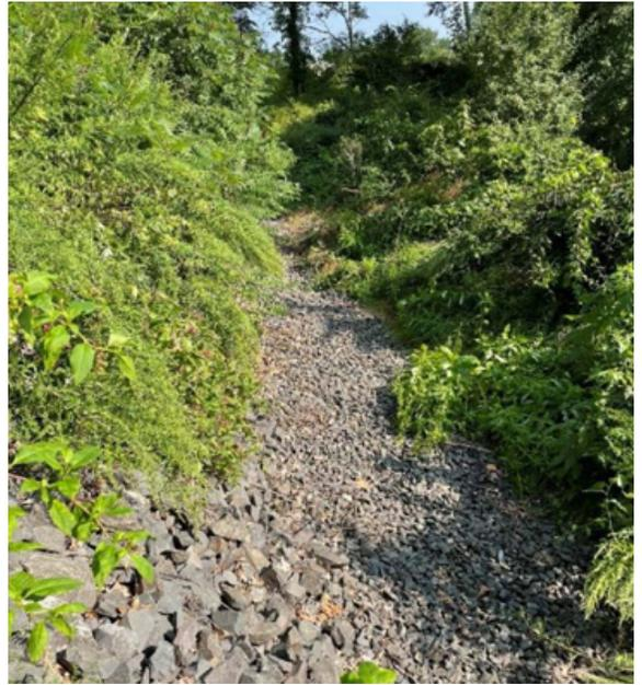
**Rock-Lined Channel:** Native plants line the sides of a rock-lined channel designed to carry stormwater to a downgradient, onsite discharge area. The vegetation helps prevent erosion while filtering the stormwater, promoting stormwater infiltration, and slowing the flow of additional stormwater entering the channel.
