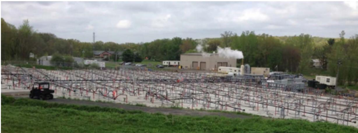
**ISTR Operation:** Thermal remediation was conducted in a 1.75-acre area in 2014-2015. The system employed more than 1,400 heaters, vapor recovery and monitoring wells. ISTR removed approximately 99.5% (nearly 500,000 pounds) of the soil's solvent contamination.
