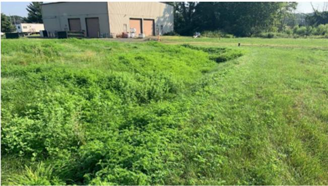
**Vegetated Swale:** A vegetated swale along the perimeter of the soil/sediment cap collects stormwater shed from the cap's surface. The swale also receives stormwater runoff from adjacent impervious surfaces or built structures, such as the former groundwater treatment building. The building now houses auxiliary equipment, controls and supplies for the groundwater extraction and solar energy systems.
