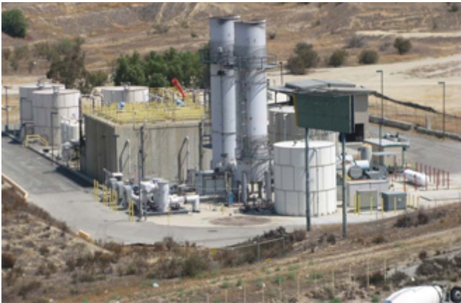
LFG Treatment System: LFG from both parcels constituting the Oil site is treated at a single facility on the relatively flat 45-acre "north parcel" where retail redevelopment is anticipated.
