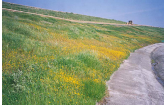
Evapotranspiration Cover: The evapotranspiration cover at Oil uses plants native to the region.
