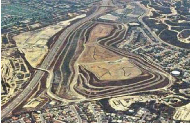
Aerial View: The Oil site consists of two parcels divided by California Highway 60, approximately 10 miles east of Los Angeles; from 1954 until 1984, this property accumulated over 38 million cubic yards of municipal solid waste.
