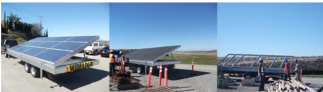
Solar Pilot Arrays: The 2012 solar pilot test deployed three self-ballasted units: one off-grid unit consisting of 12 235-watt panels and all electrical instrumentation necessary to generate and monitor electricity (shown on left above); a frame holding plywood panels (shown at center above) with added weight (an inverter, electrical instrumentation, and sand bags) to simulate both the weight and shading of a solar rack; and a bare frame unit with sand bags to simulate only the weight of a full solar racking unit (shown on right above).
