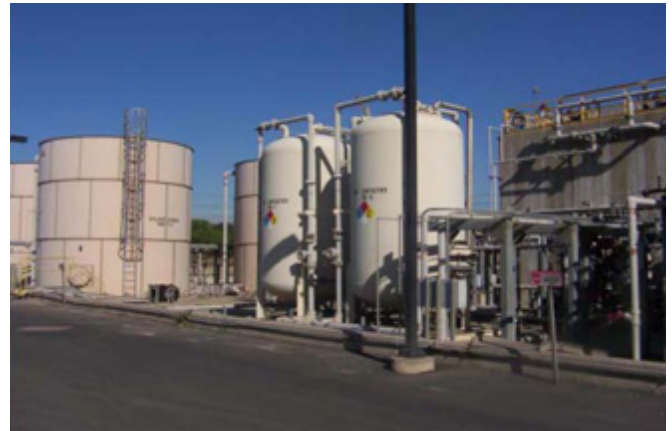
Leachate Treatment Plant: The onsite leachate treatment plant collects and treats liquids from the Oil Landfill. Liquids are collected through a system of extraction wells located along the perimeter of the site, as well as through a system of interior wells, to avoid potential contamination of groundwater and prevent contamination from migrating offsite.
