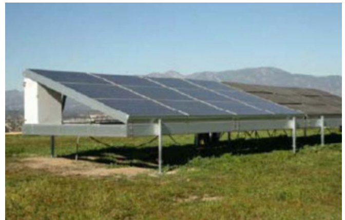
Solar Pilot Array Deployment: Self-ballasted off-grid PV panels and plywood panel units were placed adjacent to each other at Oil.
