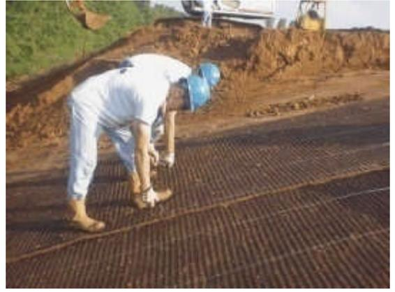
*In addition to silt fences and hay bales along construction boundaries, areas of intense stormwater runoff were lined with geotextile material and armored with rip-rap stone.*
