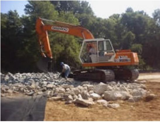
*Concrete was salvaged during demolition of flight pavement and an onsite building and sorted by aggregate size for construction use.*
