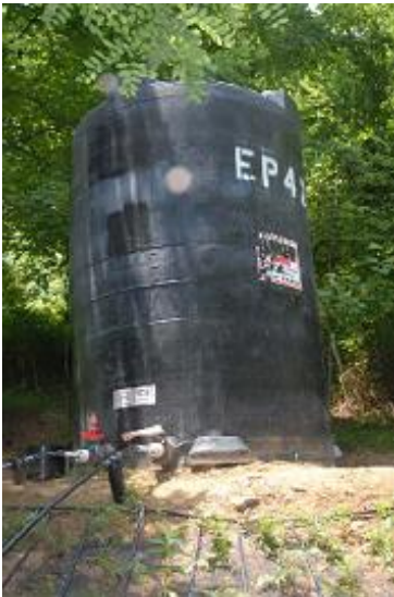
The hilltop gravity irrigation system uses a small filter and network of 1-inch PVC piping equipped with a pressure gauge.
