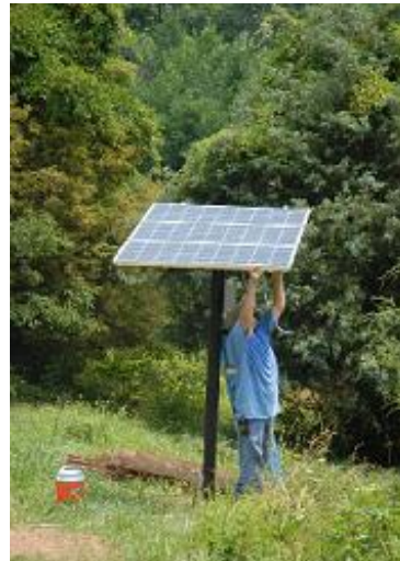
Solar energy to generate electricity for water pumping is captured by a 390-W photovoltaic array consisting of three 12-volt panels.
