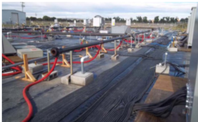
ERH Design: The ERH system covered about 26,719 square feet and contained 111 electrodes with final depths of 40, 60, or 80 feet bgs. Each electrode was set up with a soil vapor extraction mechanism. In addition, 128 shallow electrodes, also known as "puppy" electrodes, were installed where treatment was required for shallow soils less than 10 feet bgs.
