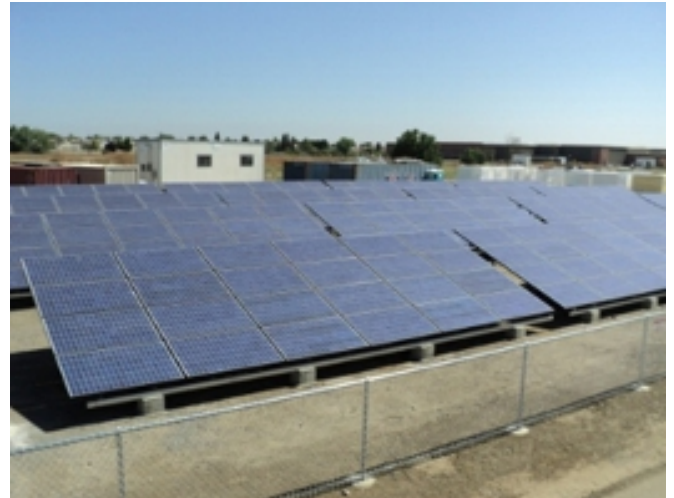
Ground-Mounted PV Panels: The 68.9-kW ground-mounted PV system installed in 2010, which consists of 336 (205 W) panels positioned on 0.5 acres of land, annually generates 101,125 kWh of electricity. System performance data are uploaded to the Internet for remote monitoring.
