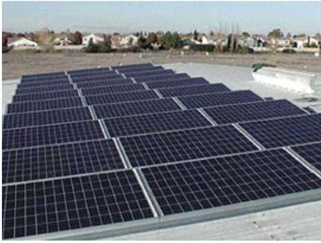
Rooftop PV Operations: The 5.7-kW rooftop PV system generates about 8,000 kWh each year and offsets a portion of the P&T system's electricity use.
