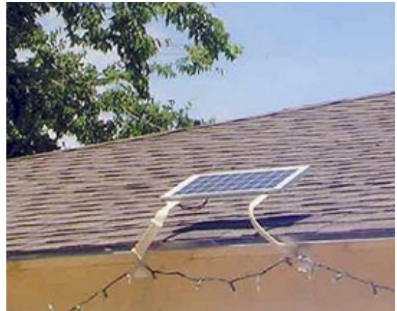
Each solar panel is installed at a 25-50° tilt with unobstructed southern exposure to the sun.
