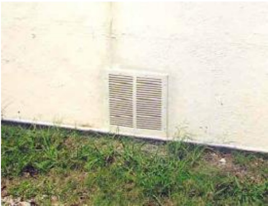
Each crawl space exhaust system vents to the building's exterior at ground level.
