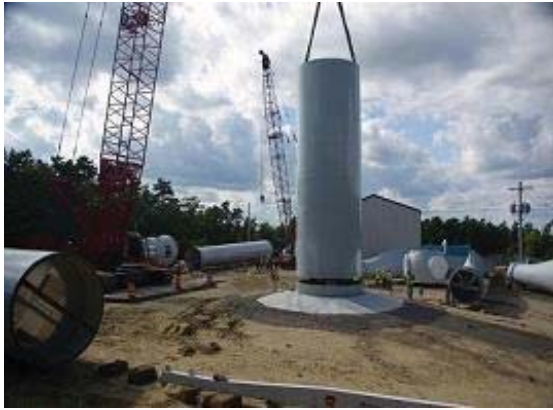
The base and sections of the wind turbine tower were set in mid October 2009.
