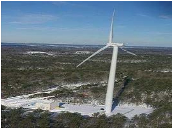
The Air Force Center for Engineering and the Environment's "FL-1500" 1.5-MW wind turbine at MMR became operational on December 2, 2009.
