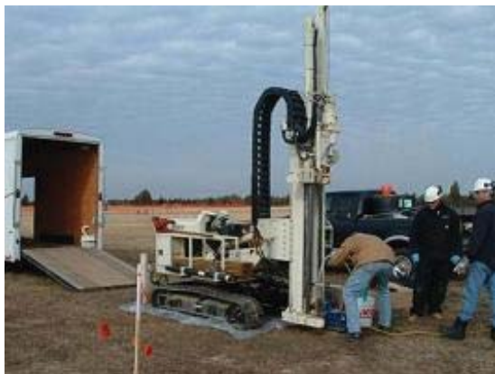
The GeoProbe 6620DT was deployed at extensive depths (up to 319 feet), eliminating the need for a larger drill rig.
