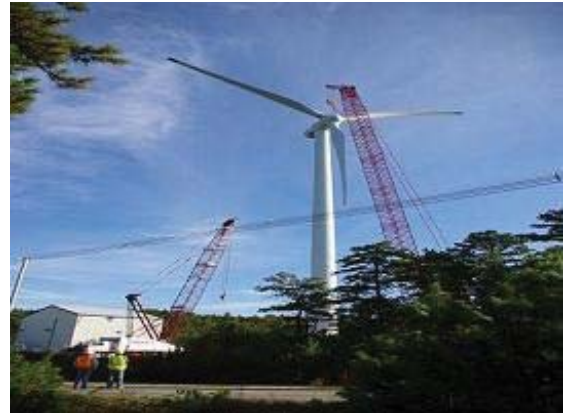
By the end of October 2009, the turbine rotor was lifted onto the tower and all construction of the MMR wind turbine was complete.
