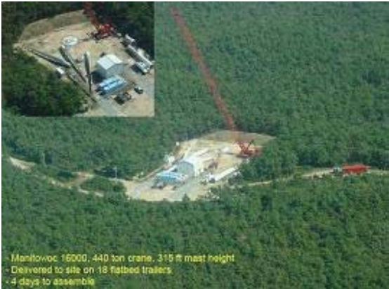
Erection of the wind turbine tower required use of a 440-ton, 315-foot Manitowoc 16000 crane, which was delivered to the site on 18 flatbed trailers and assembled near the "LF-1" treatment system over four days. Construction occurred without disruption to LF-1 system operations, which include two (blue) tanks for managing backwashing water. Mobile equipment used for each P&T system includes one (red) frac tank with two carbon vessels for treating water pumped during well maintenance.
