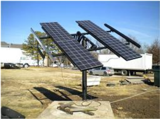
The PV system includes a passive tracking mechanism relying on the transfer of a fluid (freon), from the east side to the west side of the rack, as the sun continues to heat a reservoir (depicted above, immediately right of the rack mount) throughout the day.
