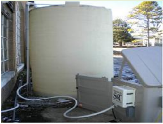
The PV system's data logger is mounted on a separate unit that houses the data management system, adjacent to two 1,500-gallon tanks where extracted water is temporarily stored for batch transfer to the onsite bioapplication trenches.
