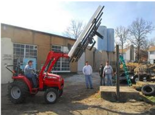
A 6-inch-diameter steel pipe serving as the PV rack foundation was installed next to a concrete slab formerly used for a storage tank, and tied to the slab to improve rack stability. Shallow bedrock at the site prevented installing the pipe to the recommended 4-foot depth.
