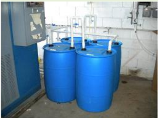
Extracted groundwater is sequentially treated by GAC media contained in four vessels housed inside the existing laundry facility.
