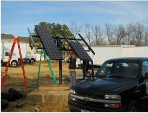
Standard construction tools were used to install each of the four 140-watt PV panels on the rack during a single day.
