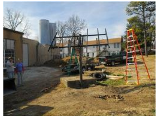
The PV system was positioned in a relatively shade-free area, due to combined effects of its distance from the onsite building and elevation from ground surface. Project designs accounted for decreasing solar energy near sunset each day, when pumping would automatically shut down, and recommencement of pumping the following day when sufficient solar energy would be available.
