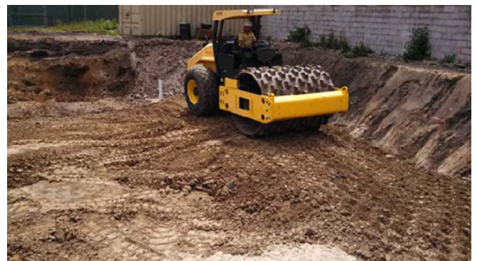
Clay Barrier Installation: Approximately 2,780 tons of clay, including 3 tons of bentonite, was compacted through use of a roller deployed in multiple rounds to achieve a 3-foot layer.
