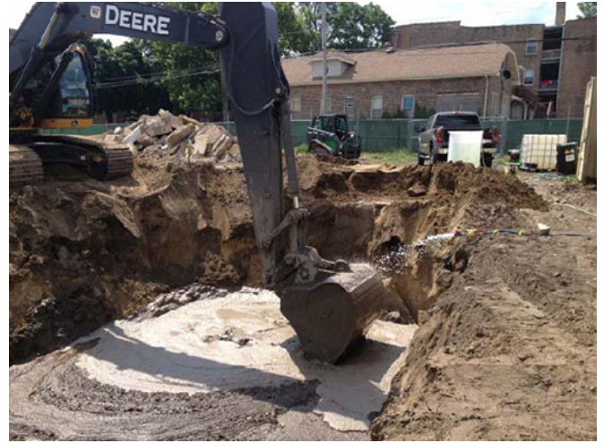
ISCO Reagent Placement: The ISCO reagents were transferred from the mixing trenches to the excavated hotspot areas where the reagents were spread into a single layer during backfilling with clean soil.
