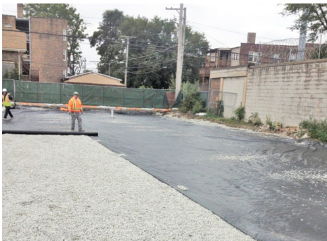
Geotextile Installation: Geotextile fabric was installed to protect the upper surface of backfilled areas and to serve as a filter around a stormwater detention basin.
