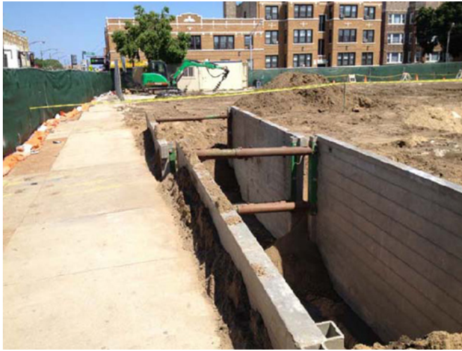
ISCO Reagent Mixing Trenches: The chemical oxidation reagents were mixed in three 16- by 16-foot trenches reinforced by steel. After mixing was complete, the steel was removed and reused onsite for purposes such as sidewalk shoring.
