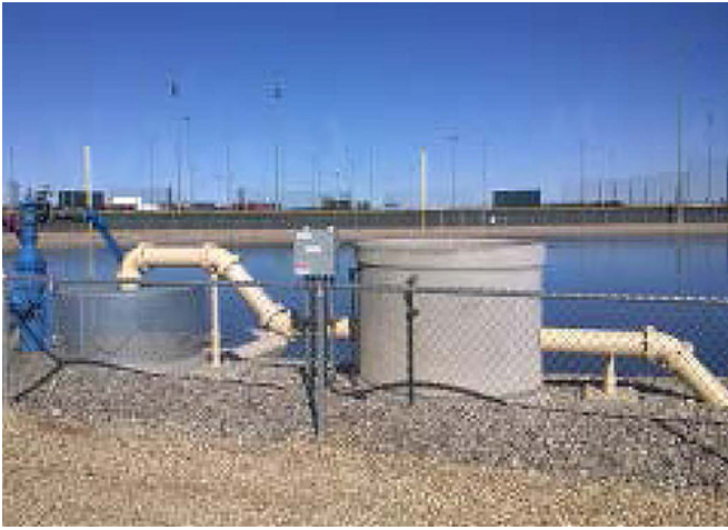
Recreation Complex Water Storage: Treated water transferred from the site's south area is stored in a reservoir at the Goodyear Recreation Complex for onsite distribution for irrigation.
