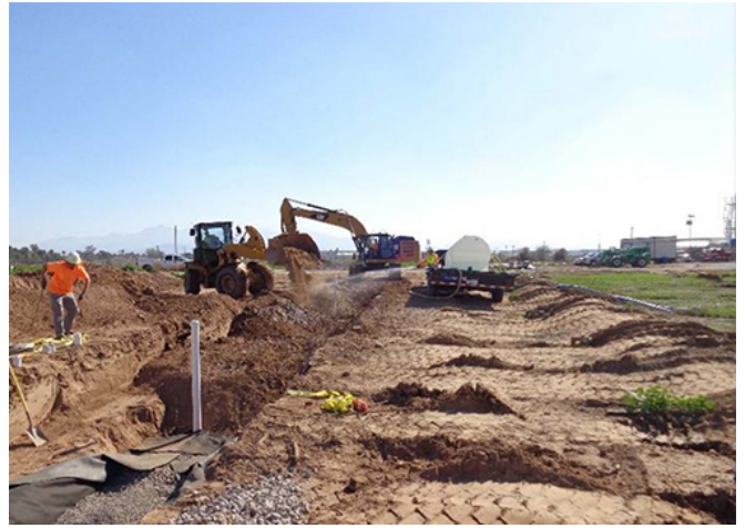
Infiltration Gallery: Two onsite infiltration galleries were installed in positions parallel to opposing borders of the agricultural plot area.
