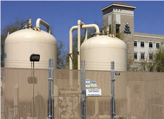
EA-05 GTS: Groundwater is extracted through one north area well at a rate of 450-500 gallons per minute and conveyed to the EA-05 GTS for VOC removal via two LGAC vessels and associated influent and effluent bag filters.
