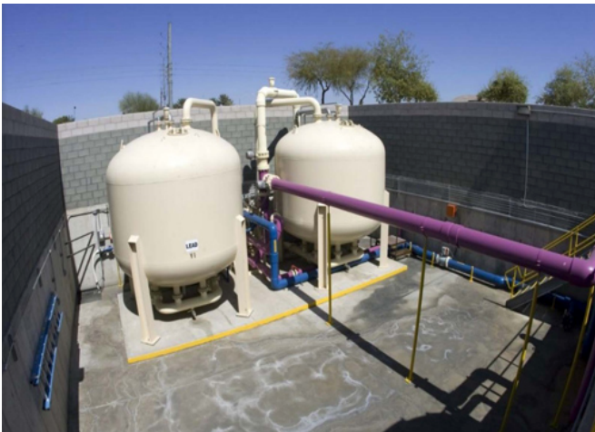
EA-06 GTS: The north area's EA-06 GTS consists of two liquid-phase granular activated carbon (LGAC) vessels for removing VOCs from groundwater that is extracted from two wells at a combined rate of approximately 625 gallons per minute.
