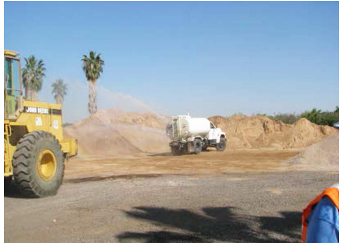
Dust Abatement: The Maricopa County Flood Control District uses a portion of the EA-05 GTS effluent to control fugitive dust throughout the county. The remainder is injected back into the aquifer through a single injection well.
