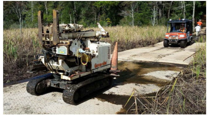
Marsh Sediment Boring: Direct-push Geoprobe equipment resting on hollow HDPE mats was used to obtain marsh sediment samples from shallow depths.
