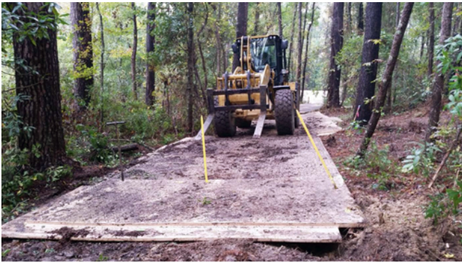
Protective Mats: Plywood sheets were placed along a defined corridor enabling machinery access to the marsh. The matting reduced sub-grade damage.
