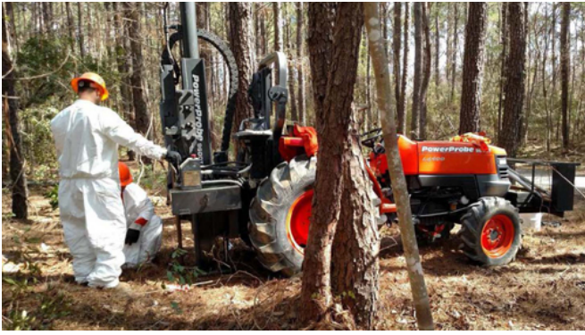
Soil Boring: PowerProbe® equipment was used to advance soil boring in wooded areas and other tight spaces.
