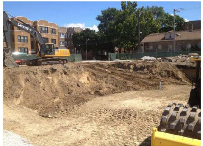
**Machinery Deployment:** Diesel fuel consumption and associated air emissions of machinery such as a 250-horsepower excavator and a 100-horsepower soil compacting roller were reduced through engine idle restrictions.
