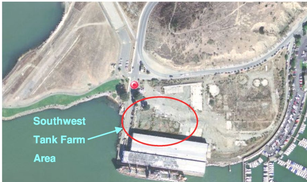
Terminal One Site Post Demolition of Tank Farms - 2004
