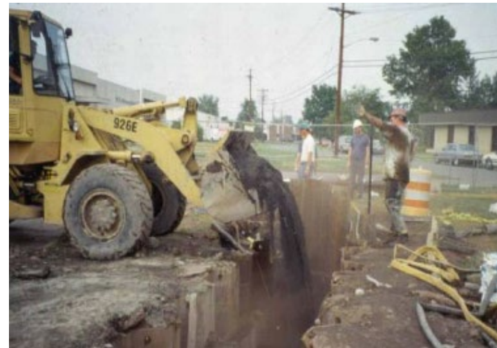
(Permeable Reactive Barrier: Technology Update, ITRC, 2011)
