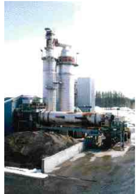
Figure 2: PCB incinerator in St. Ambroise, QC (Kroeker, 2001)
