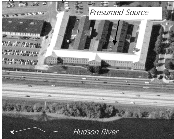
Figure 1: Building 40 at the WVA
