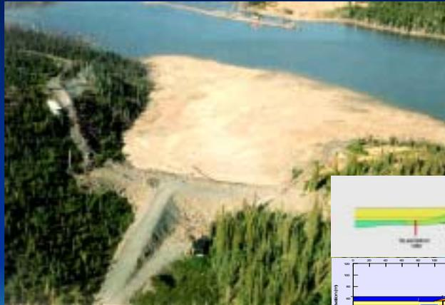
Main dam is of questionable construction. High rate of seepage.
