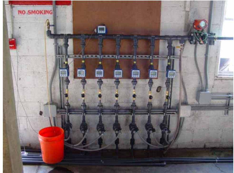
↑ Injection Manifold
