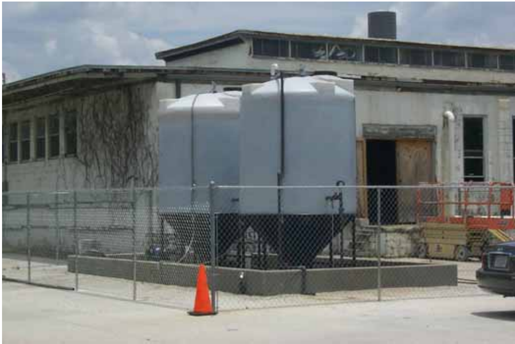
Aboveground Settling Tanks
