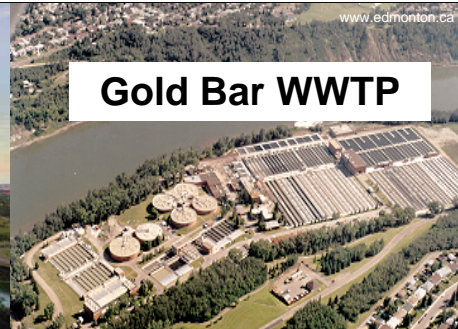
City of Edmonton
