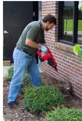
Angle beneath slab
