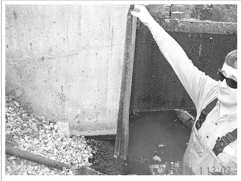
Biofouling which occurred in winter below one of the drinking water intakes in the watershed.
