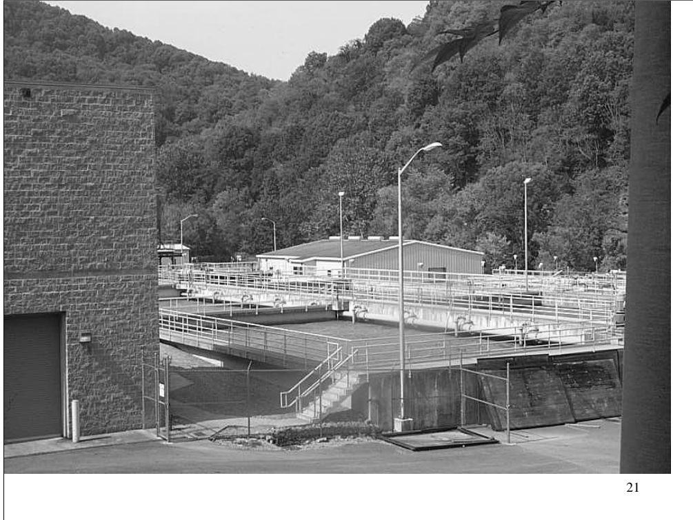
Westside Sewage Treatment Plant, Bluefield, VA serves Sanitary Board of Bluefield (WV and VA).
