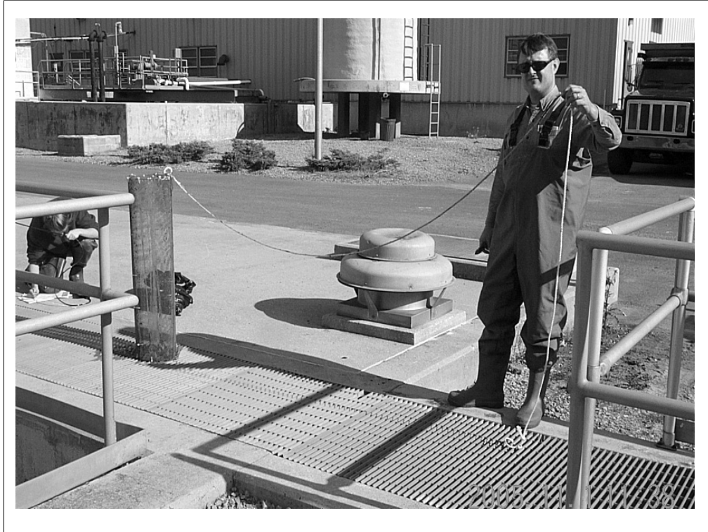
Same day retrieval of SPMD from Westside Sewage Treatment Plant chlorine contact tank just before dechlorination.
