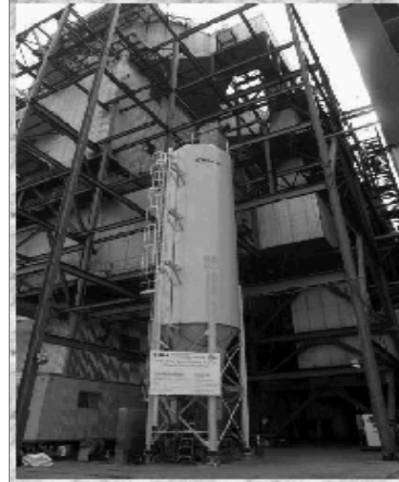
Activated carbon storage and feed system
