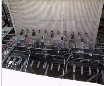
Activated carbon injection system
