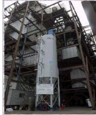
Activated carbon storage and feed system
