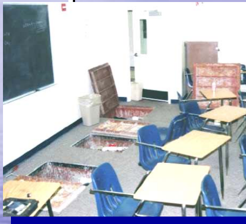
Injection Well Vaults
